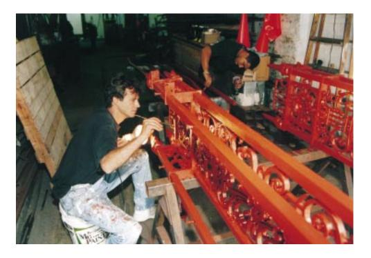
The 2001 restoration project included repairing the wrought-iron fence that surrounds the Fifth Avenue Garden. After being stripped down to bare metal, the fence was hand-painted with a rust-inhibiting primer before two coats of black paint were applied.
