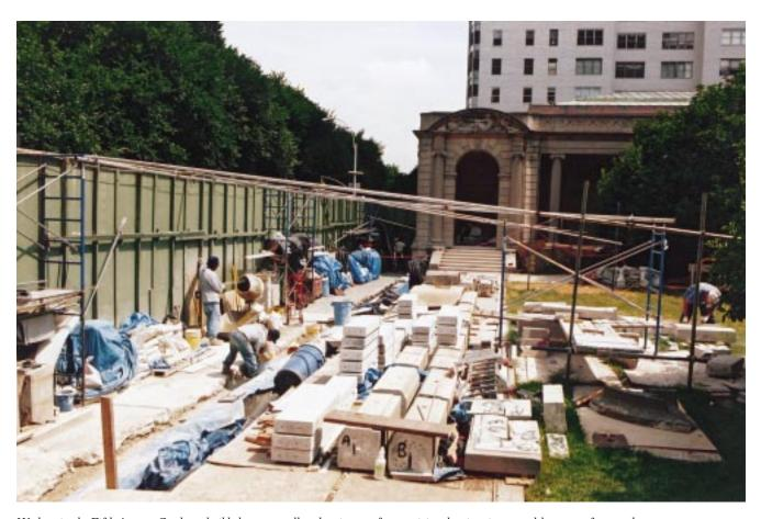
Workers in the Fifth Avenue Garden rebuild the stone wall and stairway after repairing deterioration caused by years of water damage. Whenever possible, original stones were recarved to remove damaged surface areas, then rebuilt into the repaired structures.
